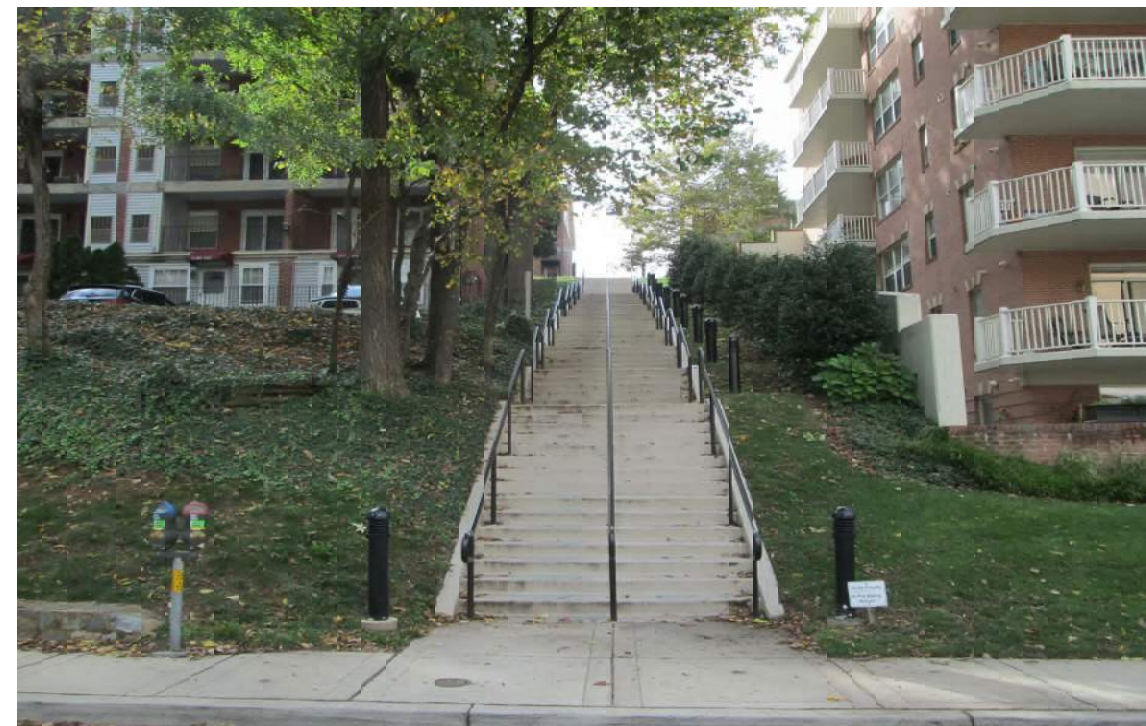
EXISTING STAIR CONNECTION TO COLONIAL TERRACE
