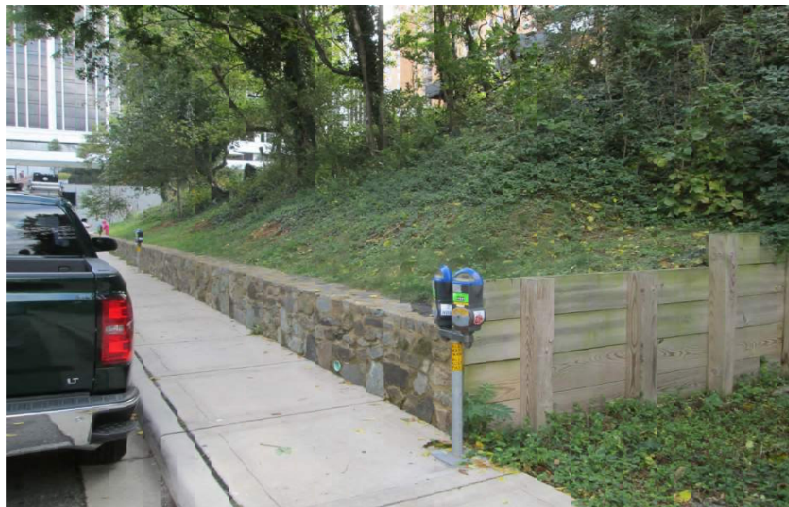
EXISTING WALLS AND SLOPE
